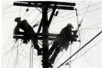
CROSSED WIRES are untangled by crews who mounted moving poles to keep phones operating.
