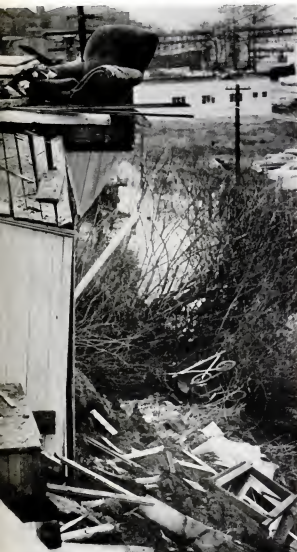
ABANDONED CHAIR remains after a bulldozer pulled down top story so it would not fall on road.
