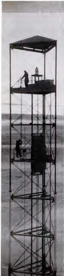
CLIMBING TOWER , the men mount ladder for last 21 feet. An elevator takes them up to that point.
