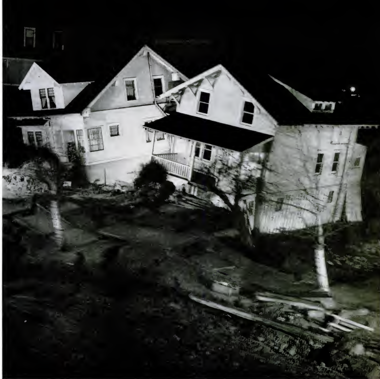
A LONG TIME EXPOSURE TAKEN ON FIRST STREET IN ASTORIA SHOWS EARTH, TREES AND PAVEMENTS SLIDING PAST PRECARIOUSLY TEETERING HOUSES
