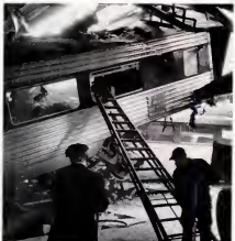
UPENDED , the rear of the first car broke through station wall. Laddler was used to get passengers out.
