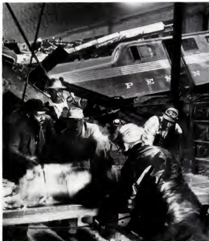
RESCUE WORKERS , right after crash, work in the baggage room below concourse where the
