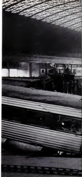
WRECK OF THE FEDERAL SPANS UNION STATION'S
