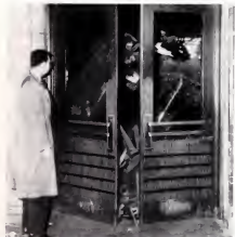
NUDGING A DOOR , a highlight on nose of the tilted engine pokes into the station's waiting room.
