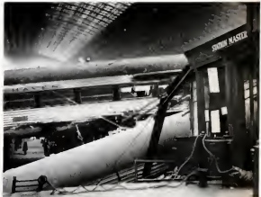
WRECKING OFFICE of the stationmaster, the first car (foreground) sank in hole made by engine.
