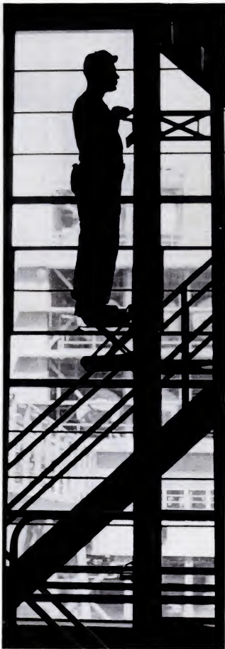
MAN-LIFT carries a workman from floor to floor in sugar refinery. Buildings, designed by H. K. Ferguson Co., are of bluish brick to reduce sun glare.
