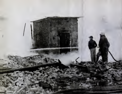
VAULT STILL STANDS on morning after the fire, although bank building around it is completely destroyed. Ruins smoked and repeatedly burst into flame for three days.
