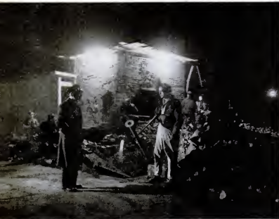
VAULT IS GUARDED by volunteers. Heat had warped lock mechanism so that vault could not be opened immediately. No one knew whether contents had been destroyed.
