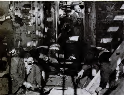
VAULT IS OPENED and bank officials find valuables intact while carpenters put up a temporary structure around vault. The bank was back in service 48 hours after fire.
