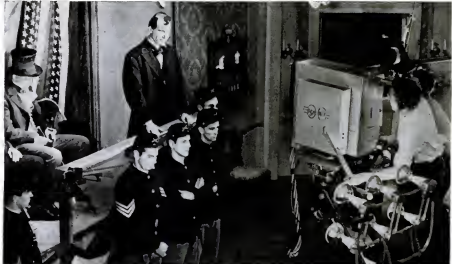
● TELEVISION NOW. With NBC, television is an actuality. Presented week after week by its New York station WNBT, programs of visual entertainment, news and public service are regularly being viewed. Here, Robert Sherwood's "Abse Lincoln in Illinois" is being televised—a production hailed by the theatrical trade paper,
