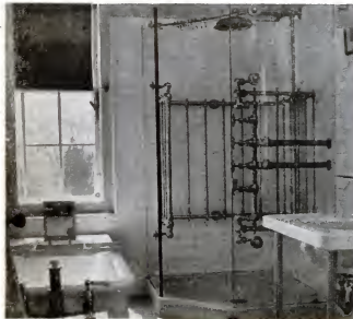
BATHROOM is old-fashioned but utilitarian. Shower (right) throws water from every angle. Mirror on the tub is specially rigged for shaving in the bath.
