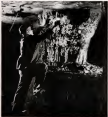
PILLAR OF COAL , a relic of old vein, is one of many on which some areas of the city still stand.
