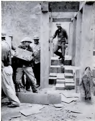
THE DANGEROUS TASK of assembling charge begins as workmen carry 100-pound blocks of TNT from loading chute to growing pile at the bottom of the excavation. Final charge was set off electrically from a trailer a mile away.
