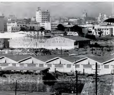
▲ MANILA has been rebuilt since its destruction during war in 1945. Warehouses fill old Spanish walled city ( foreground ). Big building in left distance is post office.
