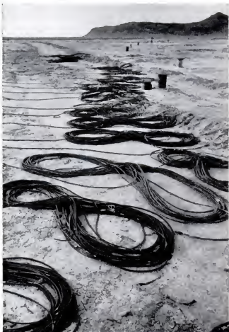
THE COILING CABLES that connected underground targets to instrument stations stretched for miles across the desert. Data recorded at these stations will indicate exact effects of blast on various types of underground shelters.
