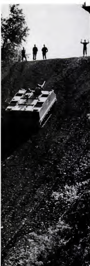
UP A MUDDY 60° SLOPE the Lifesaver climbs with little trouble. Its treads take it through mud and swamps which are unpassable to Army trucks.
