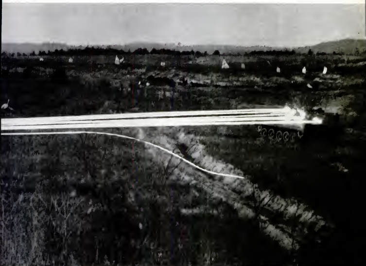
HUNDREDS OF .30-CALIBER TRACER BULLETS ARE POURED ON M-59 PERSONNEL CARRIER AT FORT KNOX, DOING NO MORE HARM THAN KNOCKING OFF PAINT
