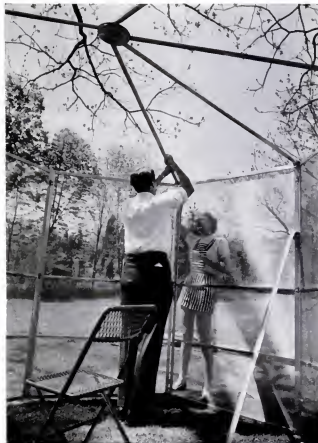
RAISING THE ROOF , the Youngs bolt roof struts to joints at top of the panels before spreading on canopy, which is anchored to struts with straps.
