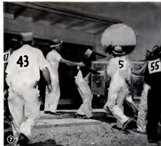
Fancy chifferoni is moved into house as construction is nearly completed. Model "family" can now take up residence. Note reflection of the crowd in big round mirror.
