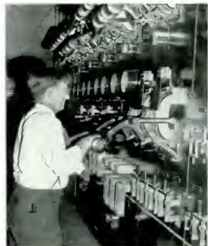
Head electrician at City Hall Generating Plant pulls switch, closing street and traffic lights as blackout signal sounds.
