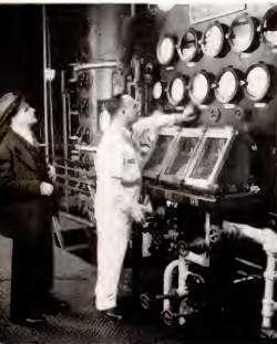
4 "In the control room of the still house, I watched the 'tail box.' This reverses the proof and quality of the distillation in process . . . diverts the first and last parts of the run back to be redistilled. . . permits only the middle run—the best—to become Old Quaker Special Reserve."
