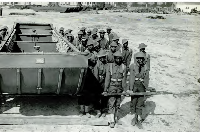
A BRIDGE, SEVERAL OF THESE PONTOONS ARE MOORED SIDE BY SIDE AND FLOORING IS RUN ACROSS THEM. WHEN COMPLETED, SUCH A BRIDGE CAN CARRY A LOAD UP TO 25 TONS HAS FOUR-WHEEL DRIVE. THE WHEELS ON SIDE ARE SPARES WHICH CAN CARRY WEIGHT IF NECESSARY
