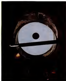
THE BATHROOM SKYLIGHT is a bomber-type Plexiglas blister. This allows natural light to enter bathroom, which in each wing is an interior, windowless room.
