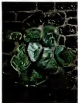
GLASS CULLETs go through the cannel coal wall, sparkle brightly on the inside when the sun strikes their outer surface.
