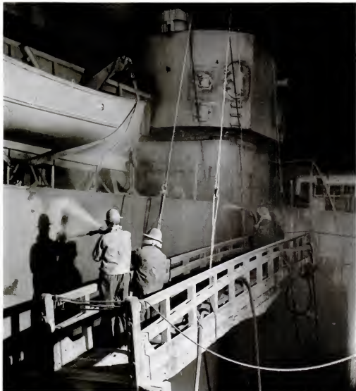
SANDBLASTING of Wiscasin's hull goes on day and night. Using a mixture of water and sharp-edged sand, not
