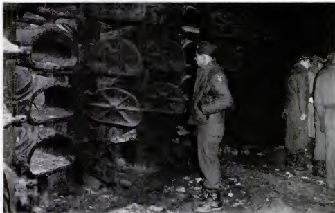
BAKERY IS USELESS because Russians took away the temperature-control equipment and other machinery.
