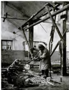
THOROUGHLY GUTTED was Teh Ho weaving and dyeing plant. Only pipes remain to indicate plant's job.
