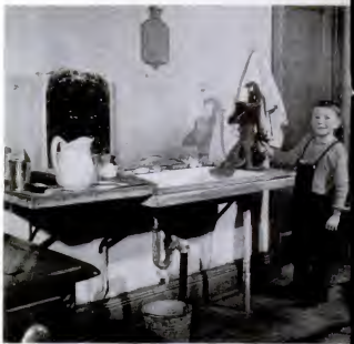
ONLY PLUMBING in the Birstengel home is pump at the kitchen sink. Birstengel says that a wife who wants electricity must "work for it first."
