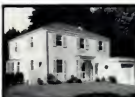
A house at Chestnut Hill, Penna., designed by Architect J. L. Cassaver for himself. Note effectiveness of Cabot's DOUBLE WHITE on brick.
