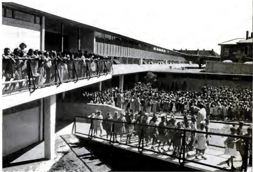
ACROSS YARD FROM OLD LAFON (REAR), PUPILS MASS AND MARCH UP INTO NEW SCHOOL-ON-STILTS
