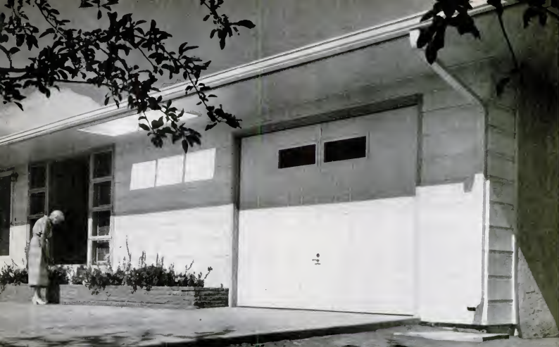
Electronic Moduflow is installed by heating dealer Charles E. Spaeth for builder McCauley, Architect Irving Coryell designs homes for the McCauley firm.
