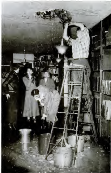
FLOOD IN THE BOOKSTACKS resulted as water pipes froze and burst in a Buffalo library after steam heat was cut off. Workers saved valuable books, damage was $3,000.
