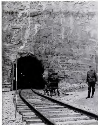
On rocky shores, huge tunnels in the cliffs supply big fixed or railway guns that can shoot across the Channel, back into France or either way along the French shore.
