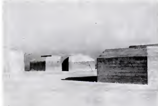
On sandy shores, where digging is not successful, these reinforced concrete bunkers, not yet finished, will hold antiaircraft or coast-defense guns of medium caliber.
