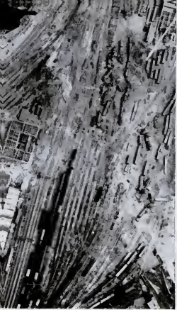
rail system scrambled. Passenger cars at right center have been blown off tracks. Bombs from another raid hit at top.
