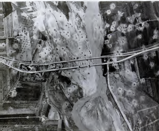
Road and rail bridges at Giulianova were bombed on March 24. Many bombs appear to be wasted, but pattern has neatly
