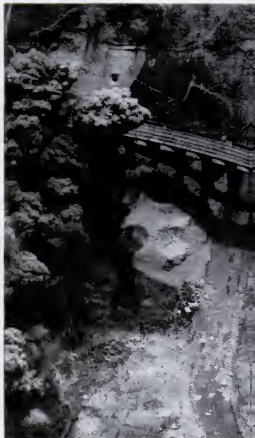
Railroad viaduct at Bucine has been knocked out by a solid hit. Other bombs land on approaches at left. One of two rail-
