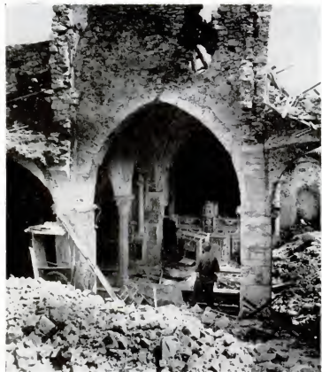
Standing in the Gothic arch of wrecked church in Castellote, an American officer inspects rubble covered interior. Castellote, which was a town of about 8,000 inhabitants in peacetime, was almost as thoroughly destroyed as Cassino by the months of allied shelling and bombing.
