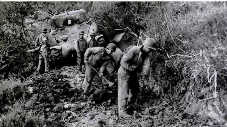
Tankmen widen lane so that their vehicles will not slip off the bank into the ditch. This lane leads to a wheatfield beyond which the infantry is waiting to advance. A few minutes later
