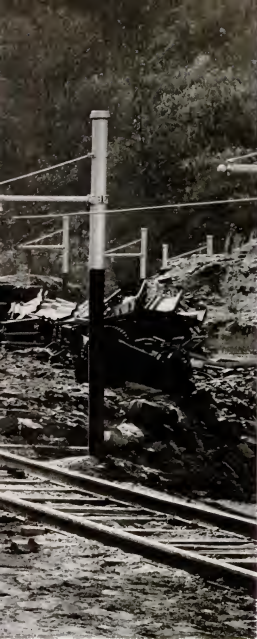
IS TYPICAL OF THE OTHER STRUCK MINES NEAR PITTSBURGH
