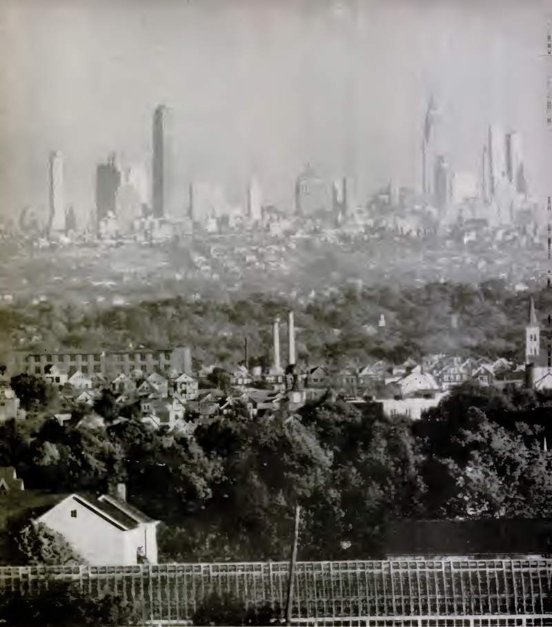
NEW YORK SKYLINE TOWERS BEHIND NEW JERSEY SUBURBS. TALL BUILDING AT LEFT IS GENERAL ELECTRIC'S. PEERING UP TO RIGHT ARE WALDORF-ASTORIA'S TWIN TOWERS.
