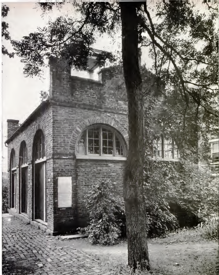
JOHN BROWN'S "FORT" WAS THIS BRICK ENGINE HOUSE OF OLD U. S. ARSENAL, NOW STANDING ON STOKER COLLEGE CAMPUS AT HARPERS FERRY, W. VA.
