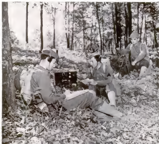
Regiment Command Post is smaller and more mobile than Division Command Post. This field set communicates with battalion. Soldier at right works hand generator.
