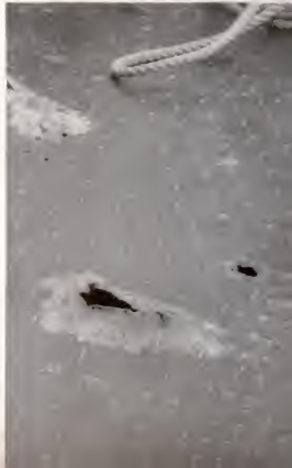
Steel plates of walkway, rent from their rivets, attest the Kearny's stout construction. The deck plating is far stronger, though lighter,
