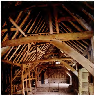
"MAYFLOWER'S" BEAMS now support a barn near London. This use of old ships' hulls was common in the 17th Century. Though the
