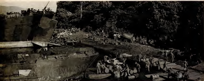
Heavy supplies are unloaded from an LCI (foreground) and an LST. Steel matting is being placed over beach to provide
