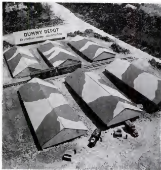
Dummy depot, with real rail line, is located near real advance depot to throw off enemy reconnaissance. Even the model trucks here are fakes or purposely disabled ones.
