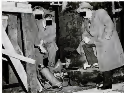
Two 2,000-gallon stills and other equipment, estimated by Alcohol Tax Unit officers to cost at least $100,000 to build and install, were seized in a Kensington, Pa., furniture plant. Elaborate and expensive installations like this are indicative of the huge profit to be made in illegal distilling.
