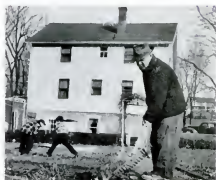
THE LA FALCE HOUSE, built on credit in 1931, is mortgaged again to pay for Johnny's college.
