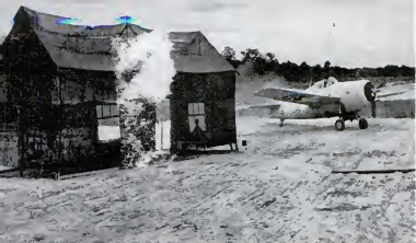
Camouflaged house is part of "farm" that conceals fighter field. It is made of fine, red wire mesh. Grumman fighter in the background is one of the Navy planes used in maneuvers.
