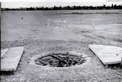
Sunken machine-gun nest , at junction of runways on field, prepares to fire on parachutists or low-flying planes. Its semi-armored top slides back after bombing attack, which preceles attempted landing.
