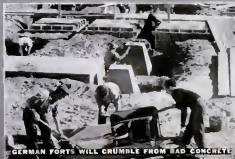
GERMAN FORTS WILL CRUMBLE FROM BAD CONCRETE
