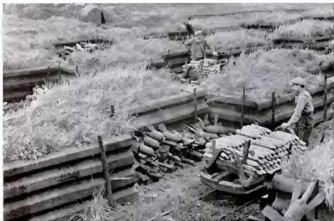
Shells and bombs are stacked in trenches with corrugated-iron walls separated by earth. Later men place each un-
