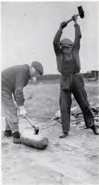
Safe to sledge-hammer was this harmless empty bomb. Workers are splitting it up for scrap. The finding company gets the metal. The Government gets the explosives if any.
