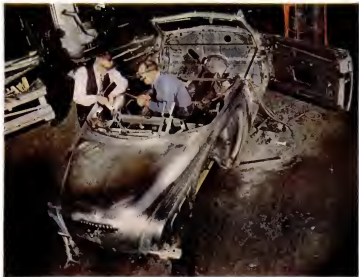
ACTUAL WORKING MODEL of car is made after mockups have been approved. Sheet metal is hammered out by hand and whole car is painstakingly put together. Such hand-built models cost as much as $30,000. They are run to death on proving ground.
