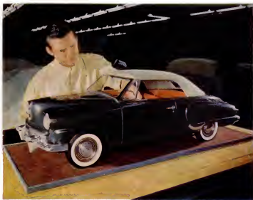
ACCEPTED VERSION of new 1947 convertible is made into a highly finished plaster model. It is completely painted and has metal trim and leather upholstery. Next step is to translate small plaster model into full-size clay model, then into a wooden mockup.
