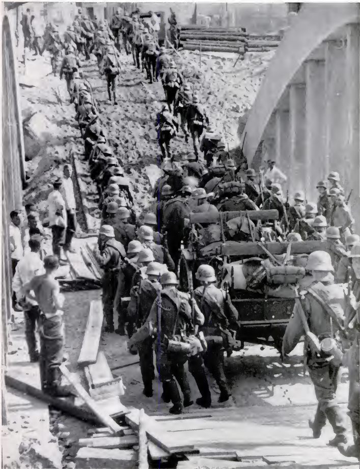
German infantry , carrying Mauser rifles, gas masks and blanket rolls, cross a half-repaired bridge "somewhere in Poland." At the side stand the Army Engineers, called
