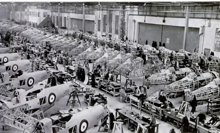
AND GLOSTER GLADIATORS (RIGHT). THE HENLEY IS A TWO-SEATER MEDIUM BOMBER WITH ROLLS-ROYCE ENGINE, THE GLADIATOR A SINGLE-SEAT FIGHTER WITH BRISTOL ENGINE
