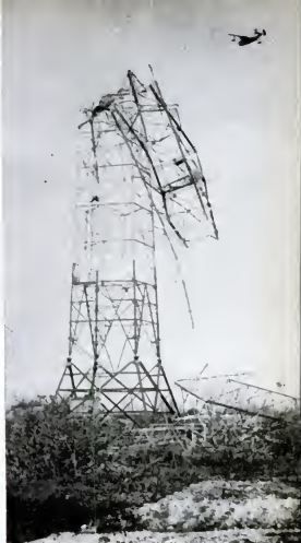
TOPS AND BOTTOMS of the island's masts and poles were cut off by storm. Above: first plane in circles toppled radio tower. Below: cross-bars suspended from wires show how wind snapped poles.
