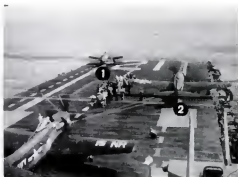
1952 TAKE-OFF is made by a drone (1) from carrier's deck under the direction of a mother plane (2). Another mother plane, already aloft, will guide it to Korean target.
