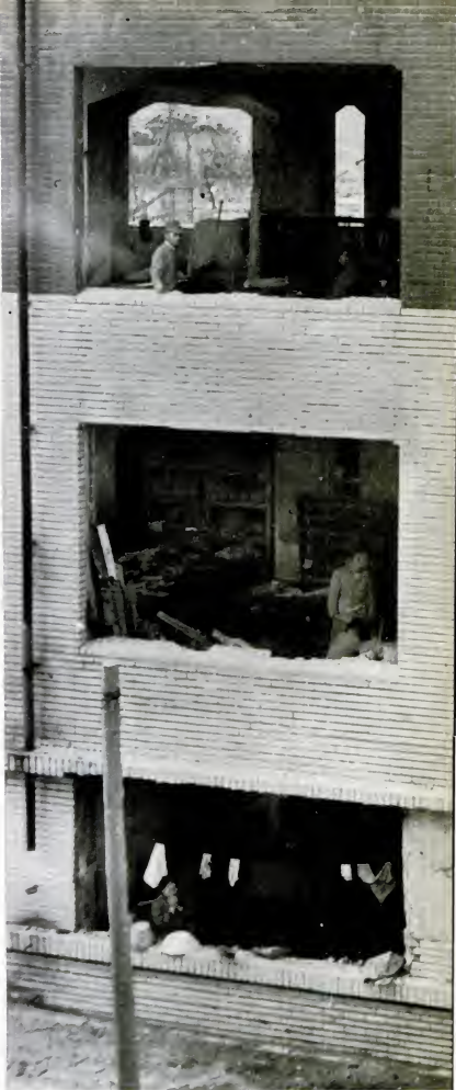
STRIPPED HOSPITAL , even window frames blown out, was soon put to use again to shelter its surviving patients on lower floor as army took over above.
