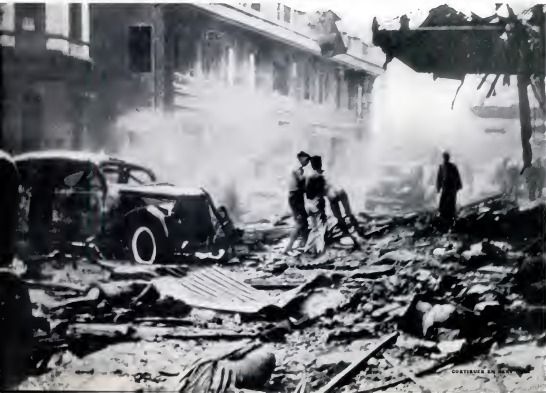
THE CATHAY HOTEL ENTRANCE AFTER BOMBING. ITS NAME ON THE MARQUEE HAS BEEN DELIVERATED; A BODY IS BEING REMOVED FROM THE WRECKAGE
