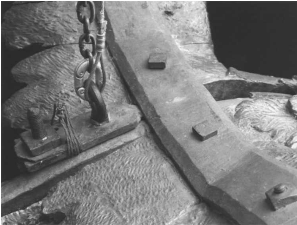
Figure 13. Detail of Eagle in Figure 1, illustrating the intersection of the three axes of its armature
