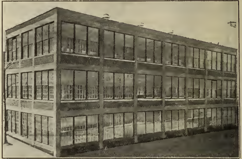
The new home of the Leather Label and Overhaul Co., Walkerville. It is of concrete and steel, absolutely fireproof. The building is practically 80 per cent. glass including a skylight roof.
