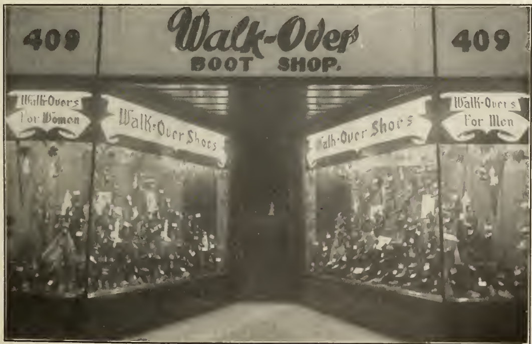
Modern store front fitted with burnished copper framework, ventilated system, marble bases and painted transparency signs. Full advantage is taken of space, glass surface and display facilities.
