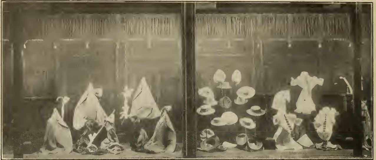
Fig. No. 2. Windows lighted with scoop reflectors placed 24 inches from centre to centre. A very open and brilliant effect is the result. See page 87.
