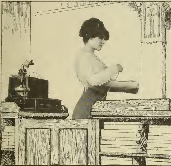
Local Station in Department Store. No. 143 Register.
