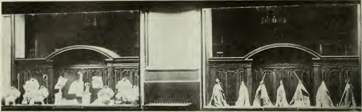
Shallow window, difficult to light, because illumination must come straight down.
