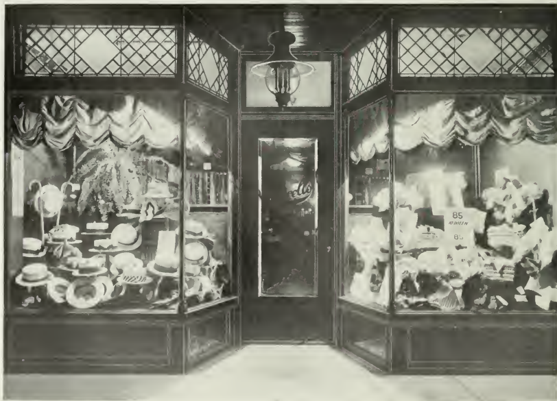
Exterior of Mr. Birrell's Store on Bloor Street, Toronto.
