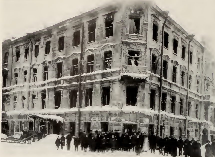
Ruins of Moscow District Police Station, Petrograd.—In many parts of the city the police defended themselves in their stations, or from the roofs or attics of houses. Whether there was shooting from the station or not, they were looted and the furniture and records burned. Where a defence was made, as in this case, the entire building was burned.
