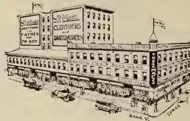
THE 2 MACS, LTD. "The Busy Store on the Busy Corner." Established 1889
