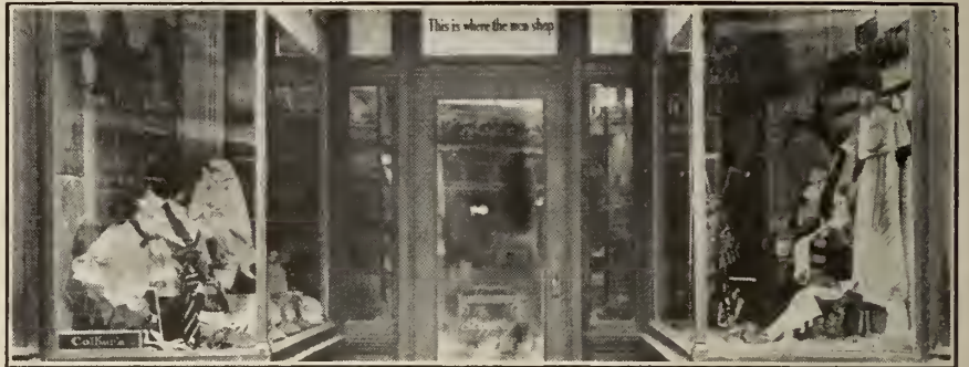
Photo showing display windows of the Collier Toggery Shop, Kingston, Ontario. Excepting for the necessary wooden framework, the entire front of the Toggery Shop is of glass, permitting unusually good lighting at all times of the day. A semi-circular leaded glass window surmounted by a bas-relief decorative finish gives a distinctly modern and well-balanced appearance to the store front. Mosaic tiling is used for the entrance.
