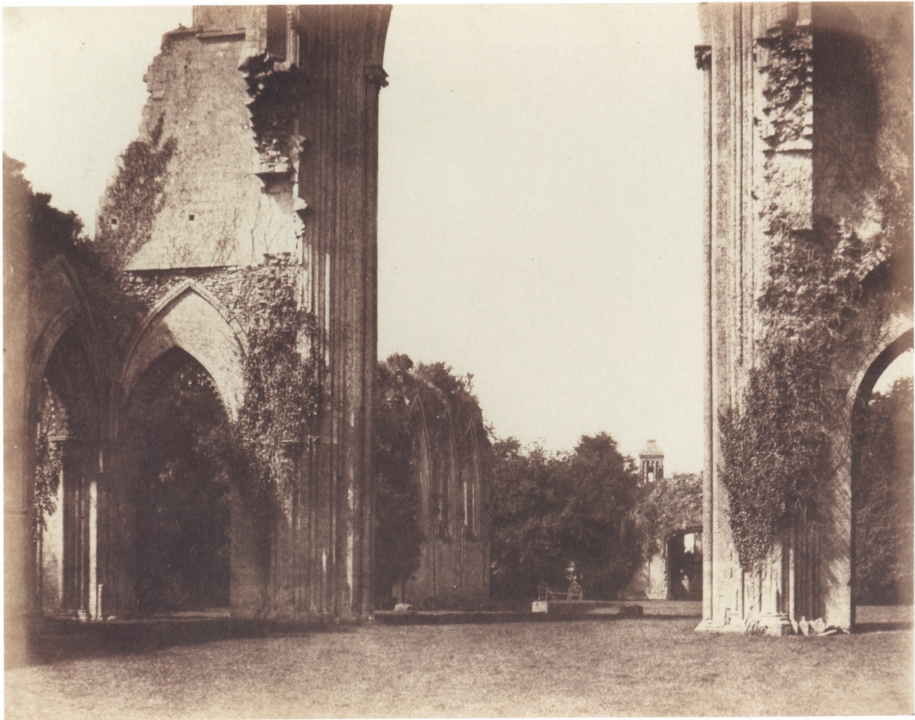
58. Alfred Capel Cure, Glastonbury Abbey, Looking West , 1857
