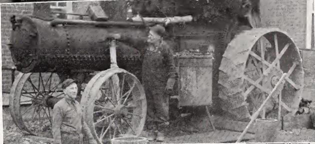
Engineer Fred Willis tunes up the 'mobile boiler' which visited us when one of the boilers in the heating plant failed to go.
