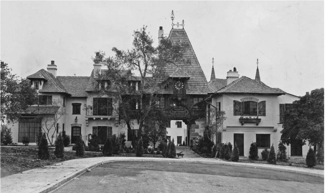
Writers got their own building, but not much respect, at the Fox Hills lot in 1932 (courtesy Robert S. Birchard).
