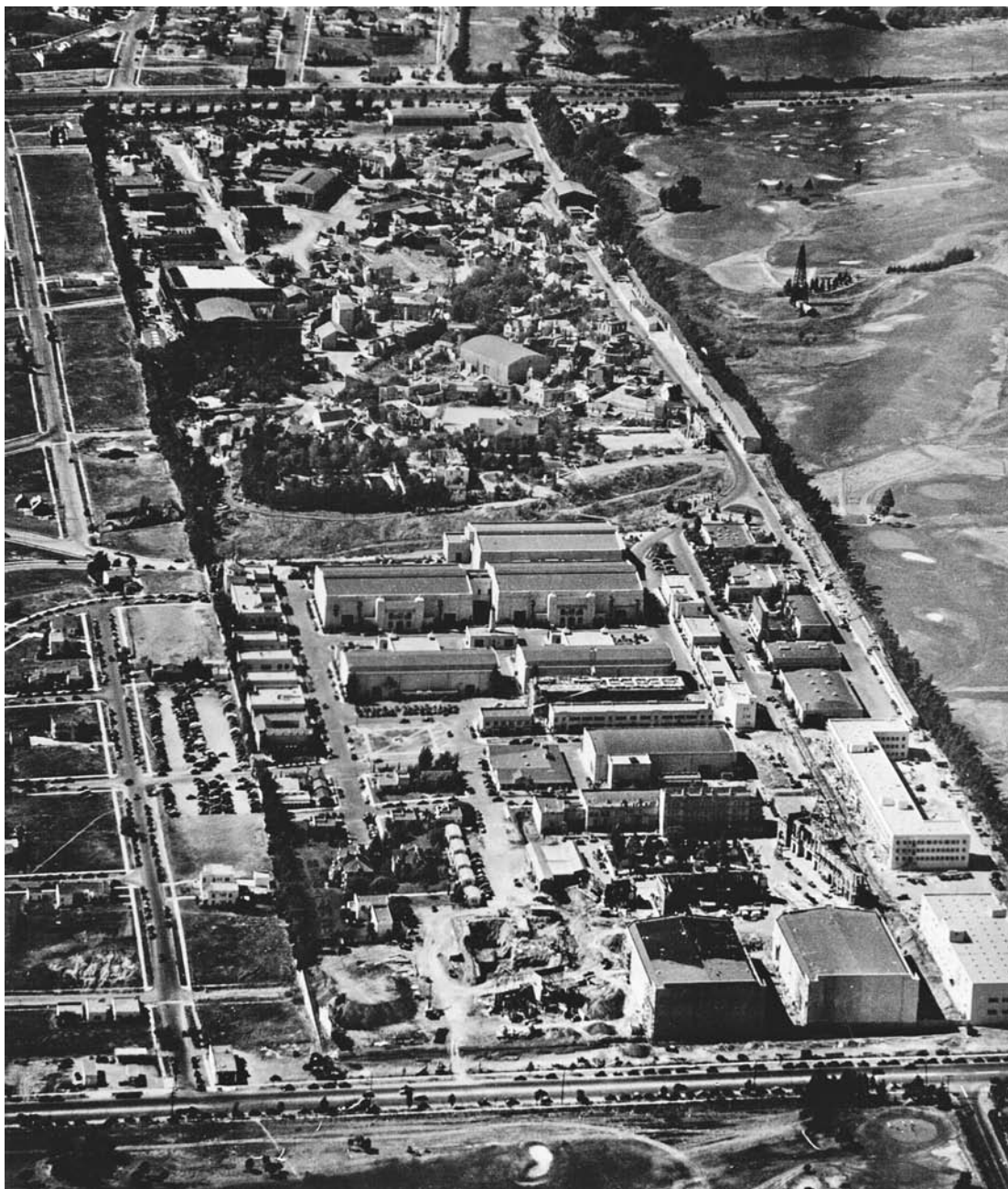
An aerial view of the Fox Hills Studio looking north from Pico Boulevard, after the merger in 1935, with standing sets clearly visible on the backlot (courtesy Robert S. Birchard).
