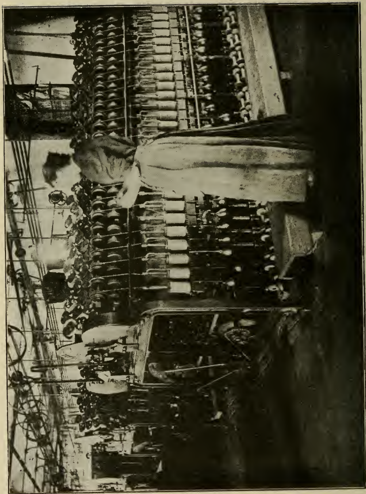
DRAWING FRAME Drawing the Roving Finer.
