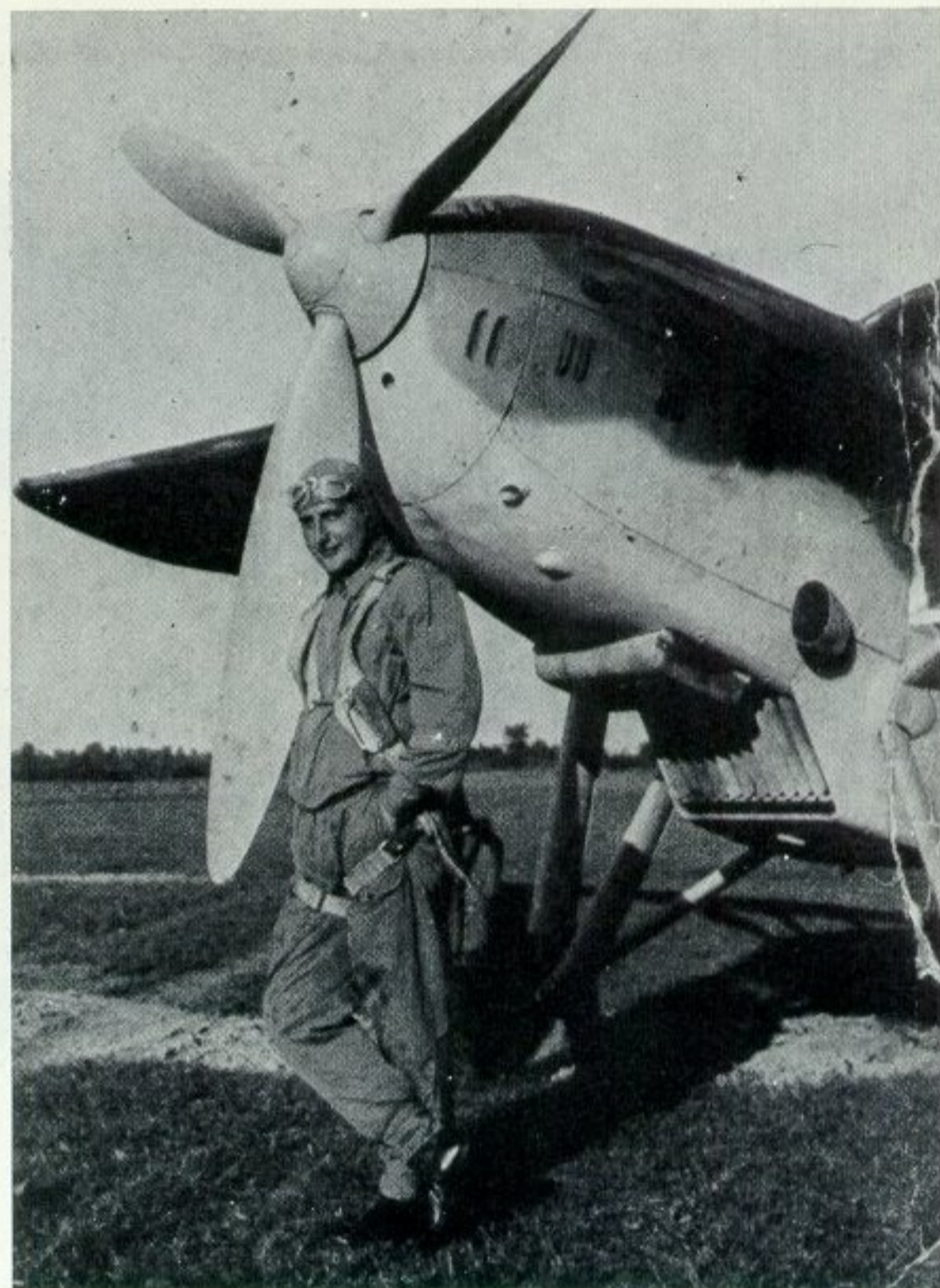
A camouflaged IK-2 with hub cannon removed and standard spinner nose cap inserted. The pilot is the former Commanding Officer of the 107th Eskadrila (34th Grupa of 4th Puk), Captain Zarko Vukajlović, who supplied this snapshot.
