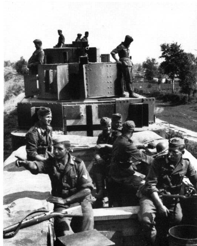
An auxiliary broad-gauge armored train (track-guarding train), manned by the 3rd Company of Railroad Engineer Regiment No. 3 in Kleist's armored unit (Southern Army Group), consisting of a Russian Type O armored locomotive (upper right), a captured two-turret artillery car, from which one cannon has been removed (lower left), and three low-board cars (with doubled walls of cast concrete or piled sandbags), manned by infantrymen, with a 3.7-cm antitank gun in front (lower right). (3 BA, 1 La).
