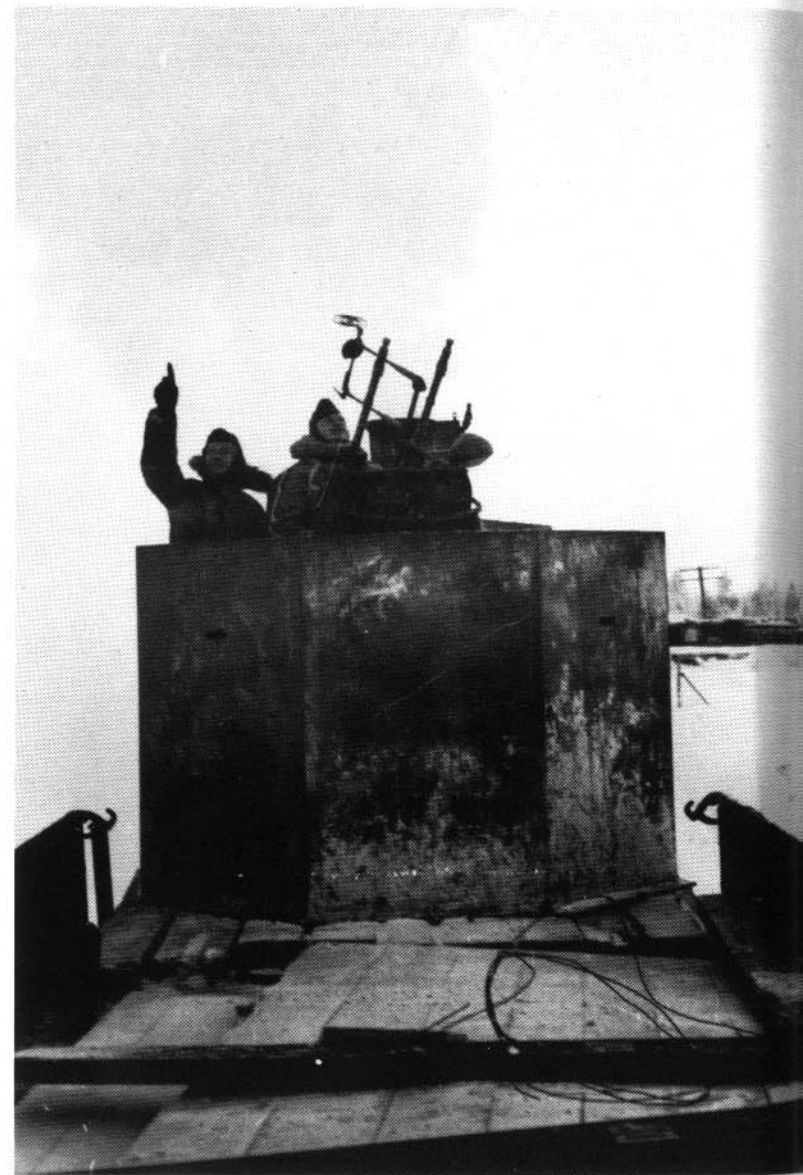
The broad-gauge armored train "Polko" was likewise powered by a Russian Type O armored locomotive. While the double anti-aircraft machine guns are housed in an auxiliary octagonal turret (upper left), the well-armed artillery car has two T-34 turrets with their effective 7.62-cm KwK. (3 x BA)
