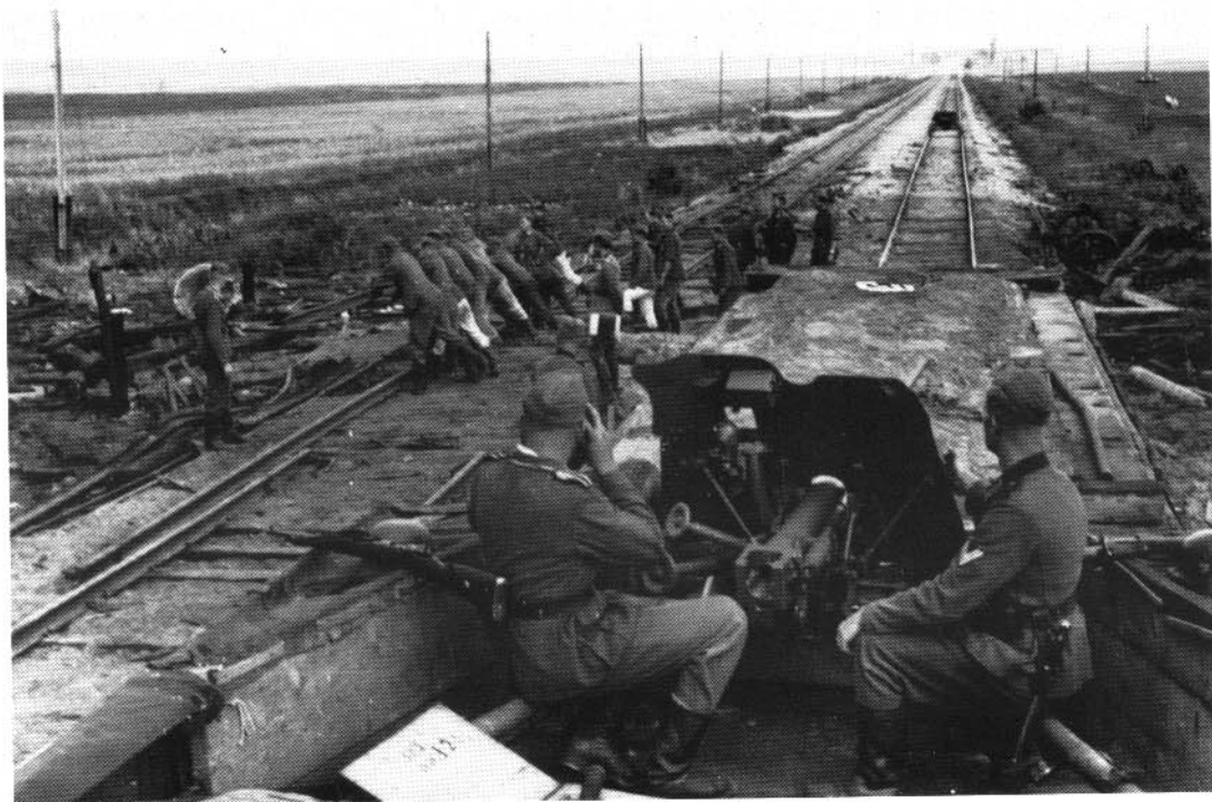
Armored trains were often called on to protect tracklaying in dangerous areas. Upper left: a track-guarding train with a 3.7-cm antitank gun guards gauge-changing work in the southern sector of the eastern front.
