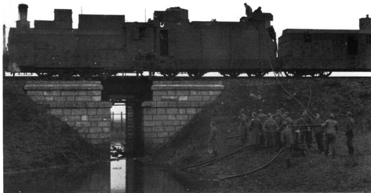
This is why the water tanks often had to be filled from bodies of water underway, using pumps brought along for that purpose. The pictures above and below show such an emergency supplying of Armored Train No. 28. (BA)
