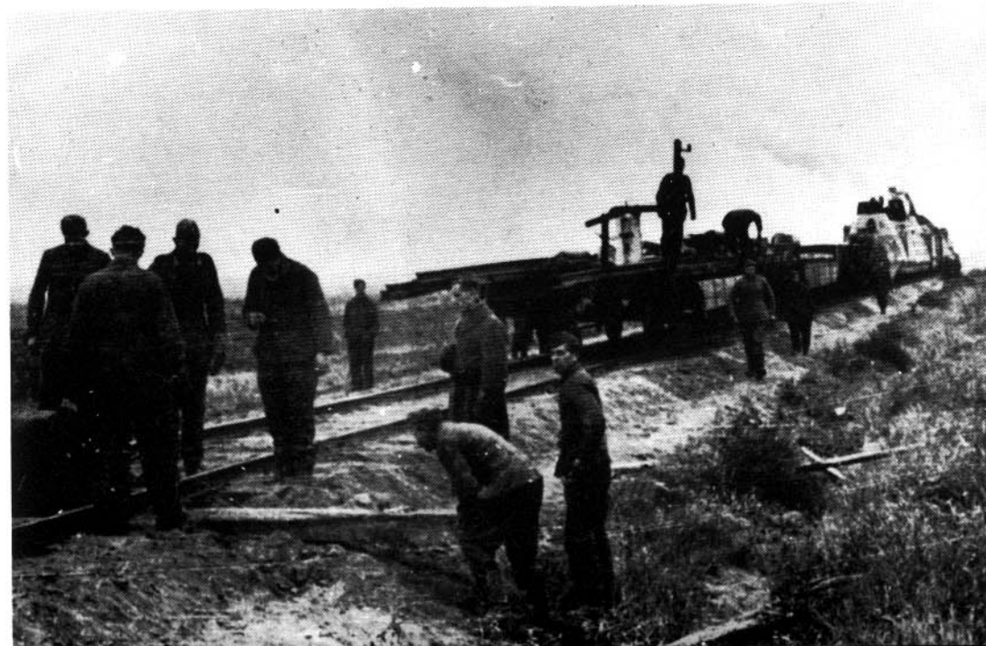
Above: Many hands had to work together to bring the rails to their places. An armored train of captured Russian cars guards the site.
