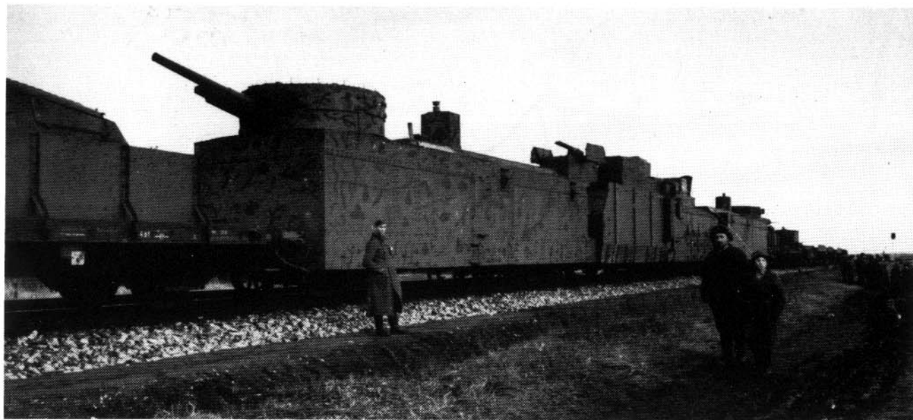
Additional pictures of the reequipped Armored Train No. 28.
